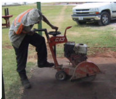
The repair process: Cut out the damaged area with a power saw. Use a pick to remove all damaged material down to the bare earth. Fill the hole with fresh asphalt, compact and smooth.
